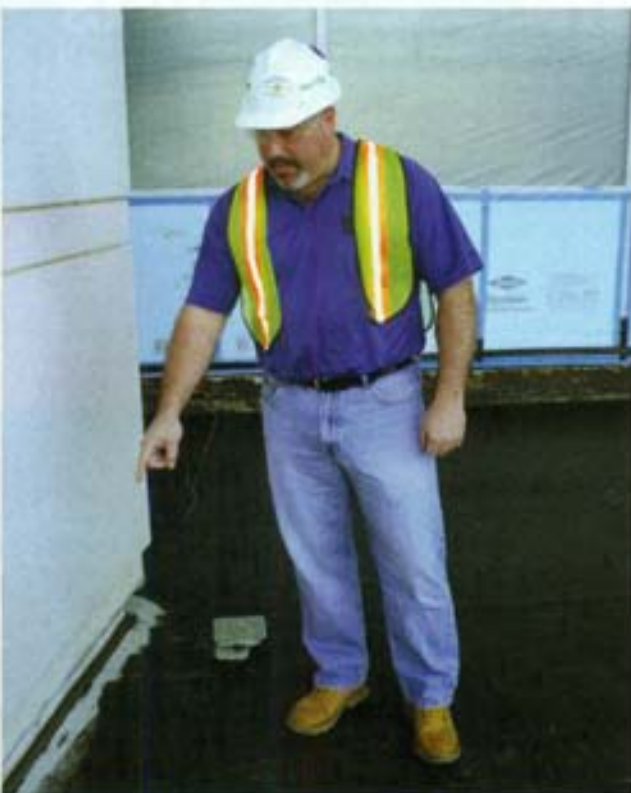
■ John D'Annunzio inspects a waterproofing project at Walter Reed Army Hospital in Silver Springs, Md. Photo courtesy of Paragon Roofing Technology.
