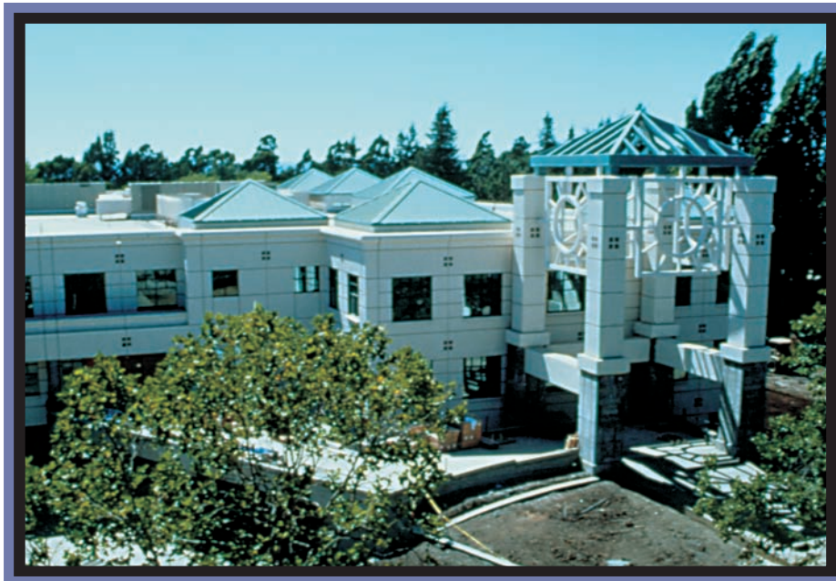
This built-up roof at the Charles Schultz Info Center of Sonoma State University, Sonoma, CA, utilized E'NRG'Y2 flat and tapered polyiso insulation by Johns Manville.
