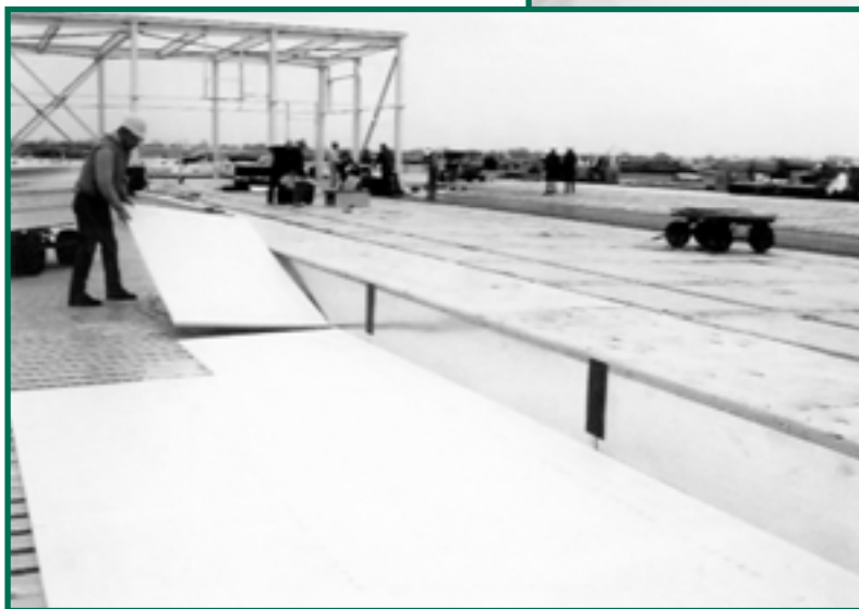
Above: Figure 4: Workers lay membrane over foam insulation at Brett Favre's Steakhouse, Green Bay, WI. (Photo courtesy Johns Manville).
