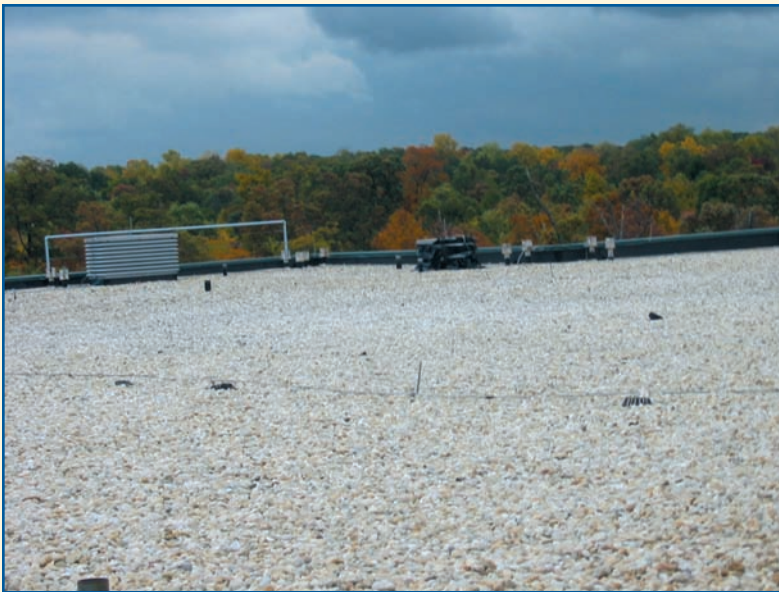
Ballasted EPDM roof.
