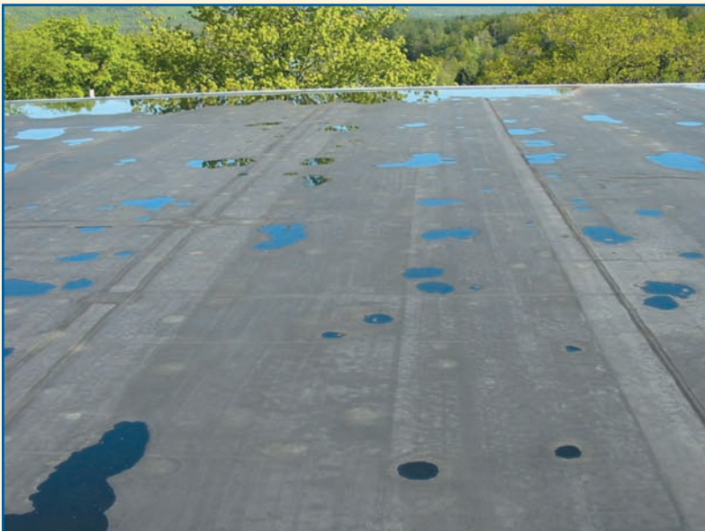
Seams on full-adhered EPDM system.
