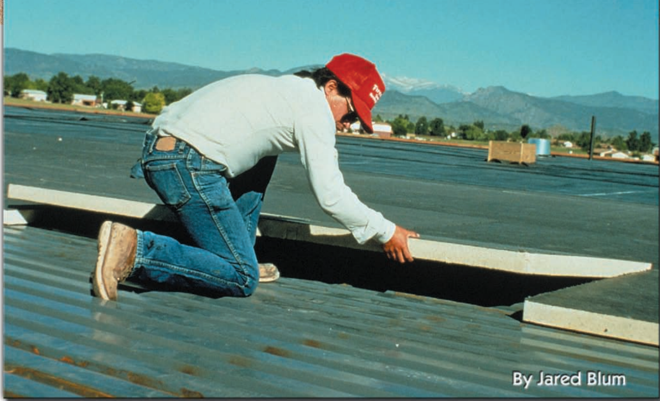
Polyisocyanurate insulation being installed on a roof deck. Photo courtesy of Firestone Building Products Co.
