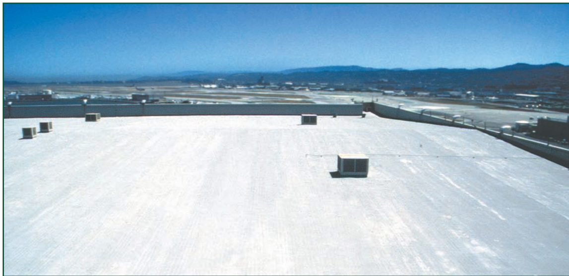
SPF systems are typically coated with light-colored, reflective coatings that utilize the albedo effect to reduce rooftop temperatures.
