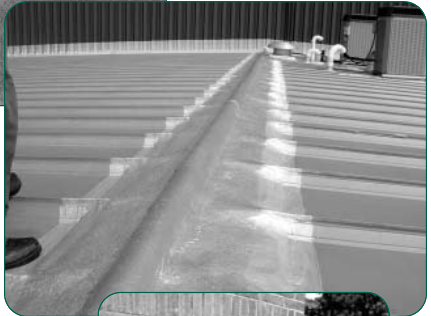
Below: Figure 2 - Metal roof expansion joint.
