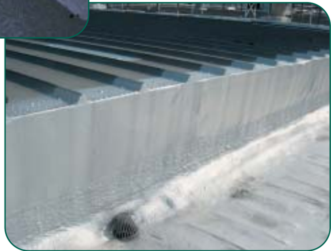
Figure 13 - SPF flashing, roof-to-wall.
