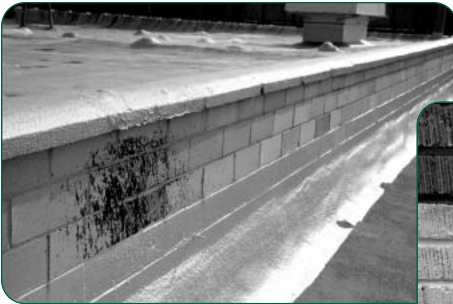
Left: Figure 6 - SPF roof and wall transition.
