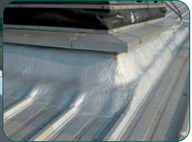
Above: Figure 12 - SPF flashing on a metal roof.
