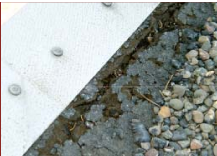
Raised edge flashing repair, before (left) and after (right).
