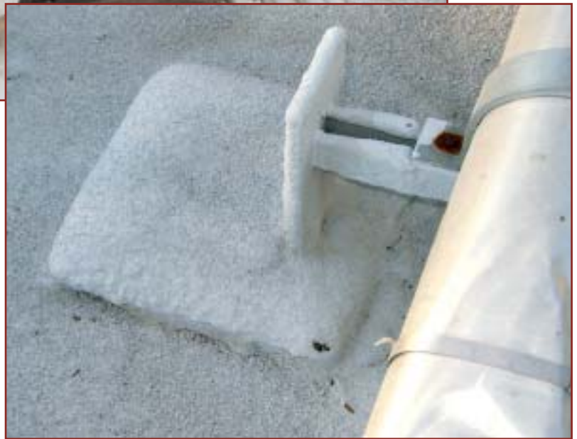
SPF and acrylic coating with ceramic granules, used to seal the pitch pan in the photo at the top.
