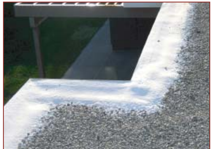
Raised edge flashing repair, before (left) and after (right).
