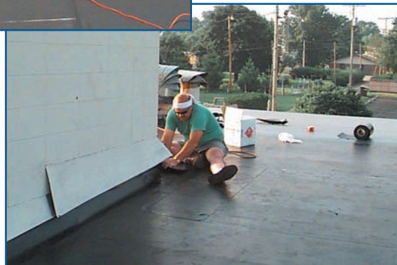
Dave Scott of Genflex detailing black TPO to wall.
