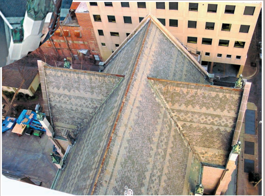
The Cathedral of St. Andrew in Little Rock, Arkansas, had worn out its black Pennsylvania slate after 120 years (below). The cathedral's new roof, left, installed by Midland Engineering in 2003, is likely to last 150 years. Vermont unfading green slate mixed with Welsh black slate and terne-coated stainless steel flashings should outperform the original roof. (Photo below by Joseph Jenkins; left photo by Lyle Bandurski.)
