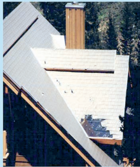
Photo 1: Damage to flat seam metal roofing.
