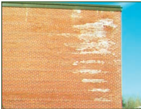
Building façade distress due to uncontrolled air leakage from the interior of a building in a cold climate.
