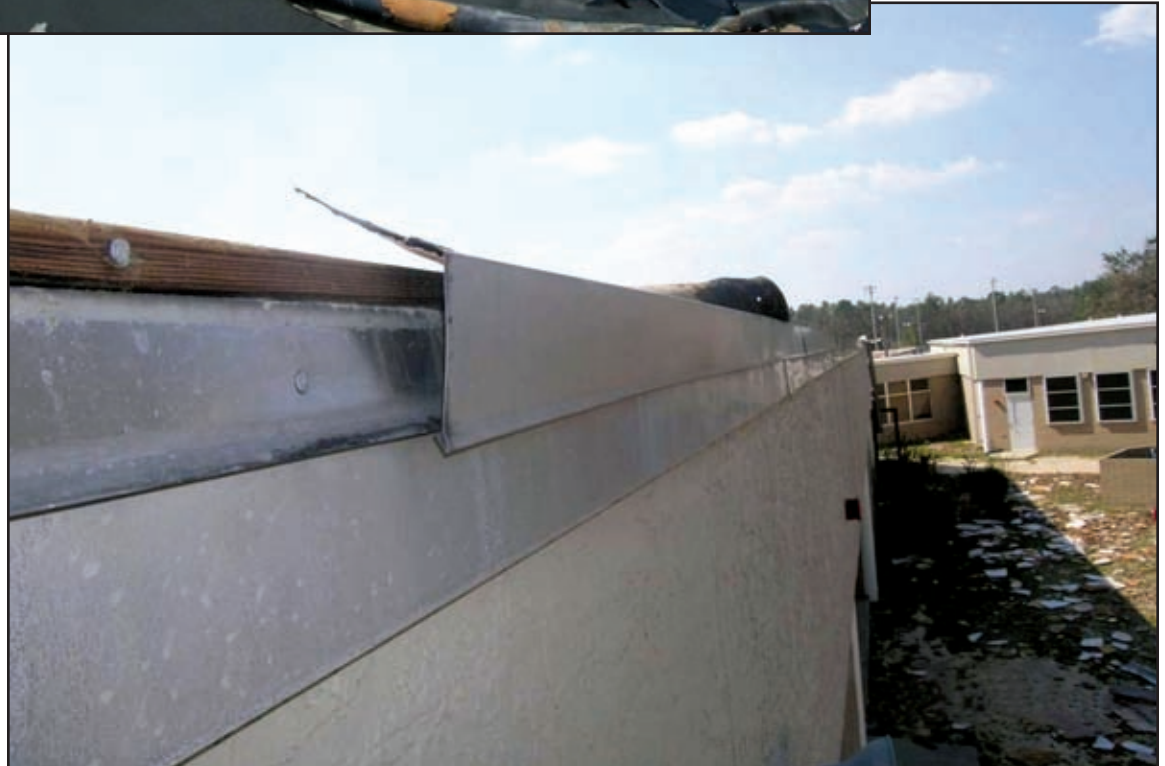
Pensacola School Building 2: Cleat deformed, edge metal lifted, membrane peeled. Cleat gauge less than currently recommended by FM Global LPDS 1-49 and ANSI/SPRI ES-1. Corrosion of roof edge fasteners contributed to expansion of edge damage into field. (Source: André Desjarlais's Oak Ridge National Laboratory report, "RICOWI and its Investigations of Hurricanes Charley and Ivan.")
