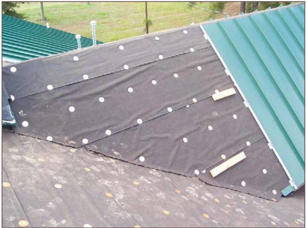
Typical wrinkled organic felt underlayment.
