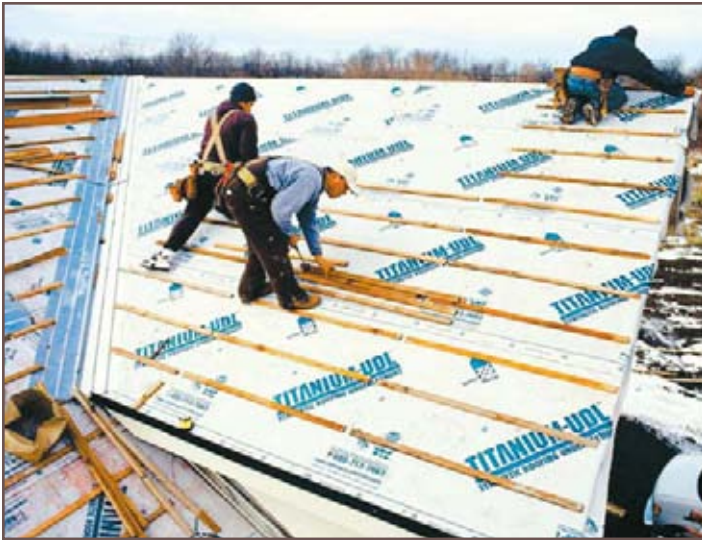
Typical synthetic underlayment installation under tile.
