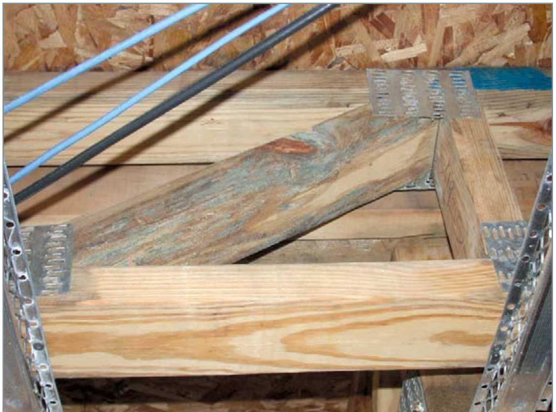
Mold on dimensional lumber.
