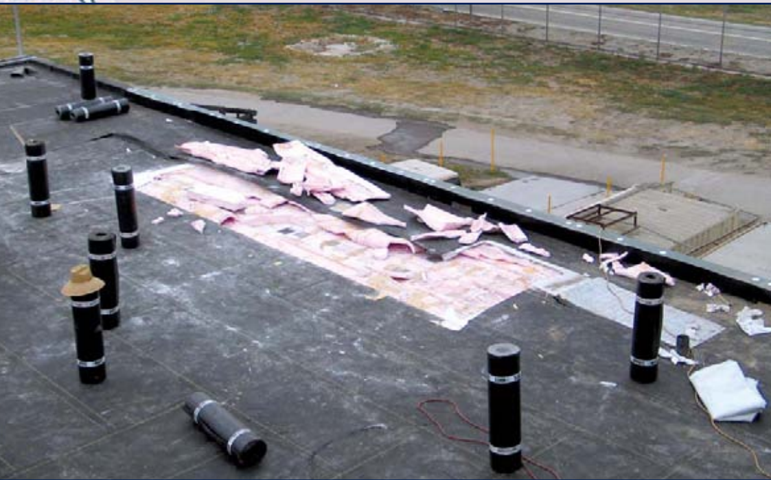
Below: The curling was so pronounced that it dislodged the 1/2-inch, glass-faced gypsum coverboard that had been adhered with urethane adhesive to the top layer of the EXPS.
