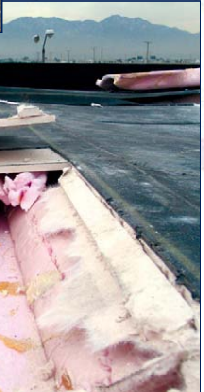
Below: The curling was so pronounced that it dislodged the 1/2-inch, glass-faced gypsum coverboard that had been adhered with urethane adhesive to the top layer of the EXPS.
