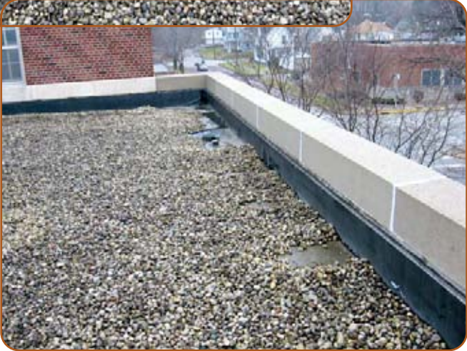
Right: Overview of roof edge.
