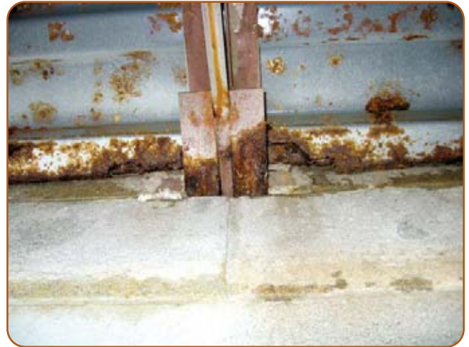
Deteriorated metal decking.
