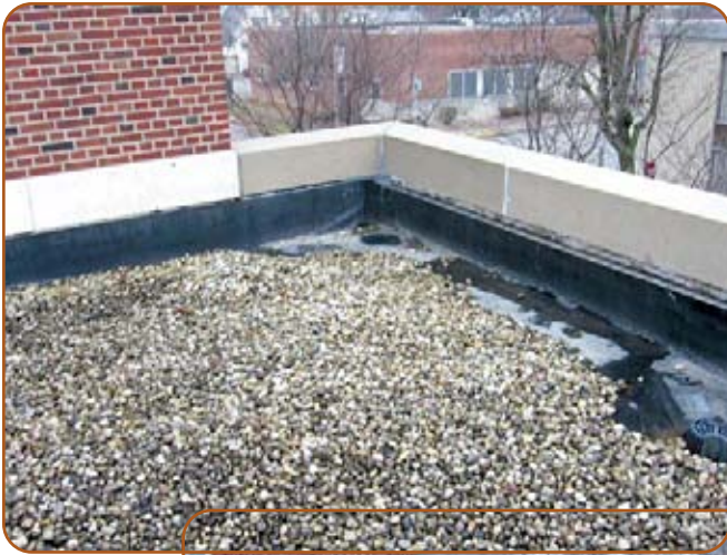
Above: Roof perimeter showing coping stone.
