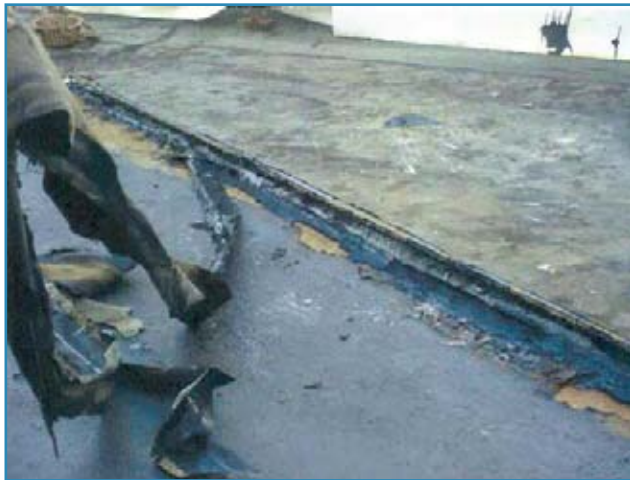
Figure 4 (above) and Figure 5 (right): Poor adhesion of primer over a wet concrete substrate. Long night seals can be sources of water under newly installed roof assemblies.
