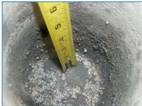
Figure 3: Core into a concrete slab to the solid pan below.
