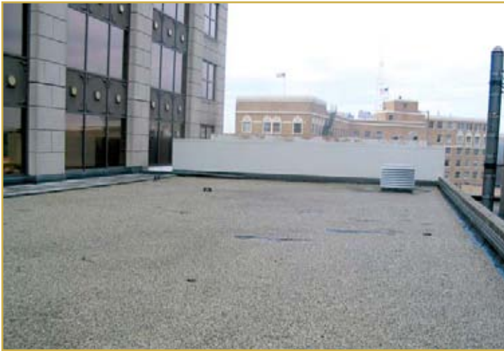
Left: Photo 5 – Overall of involved roof area.
