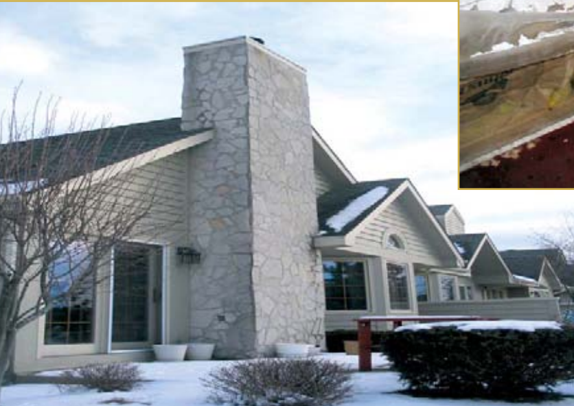
Below: Photo 2 – Typical wood-framed, stone-clad chimney enclosure.
