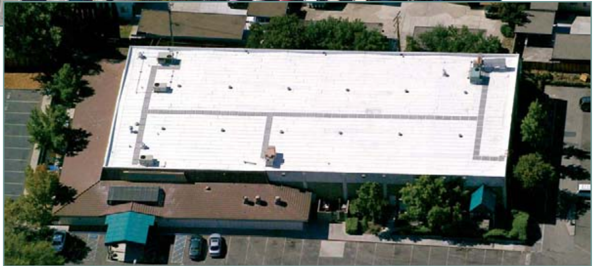
Factory-coated BUR cap sheet on Concord Center office building, Concord, CA.
