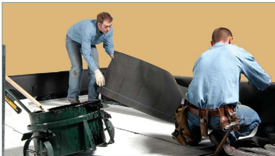
Traditional BUR installation methods work well for new factory-coated cap sheets.
