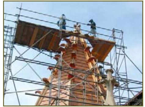
Scaffolding for difficult applications. Photo by Knickerbocker Roofing.
