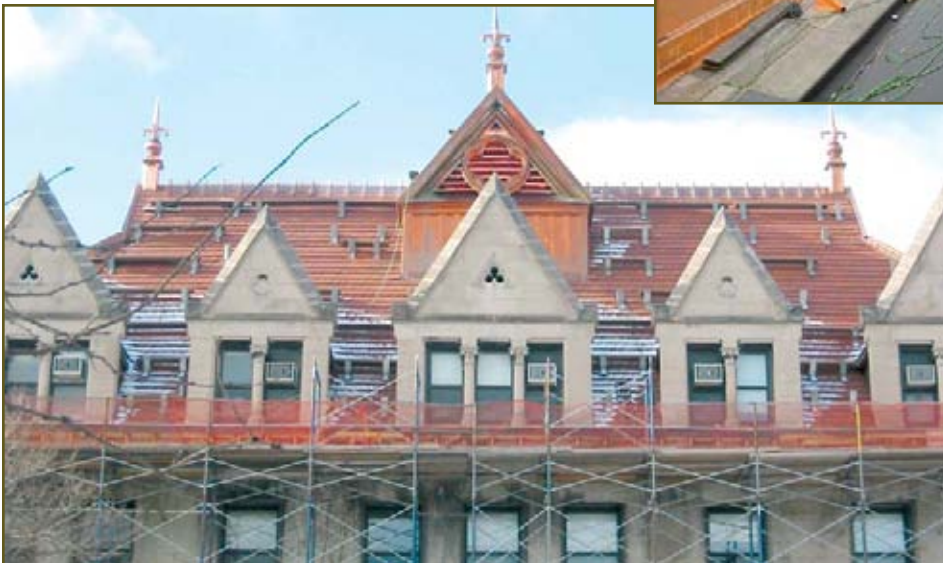
Right and Below: Scaffolding provides safety from falling debris to those below. Photo by Knickerbocker Roofing.
