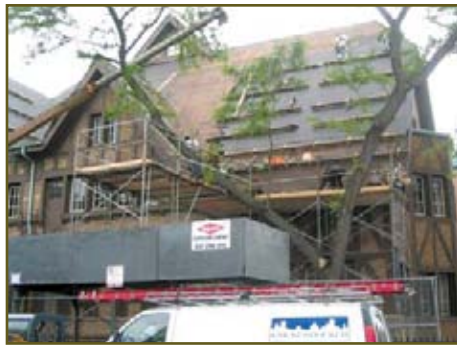
Scaffolding secures residence from damage.
