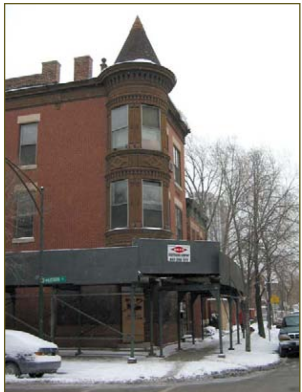
Scaffolding keeps retailers open.
