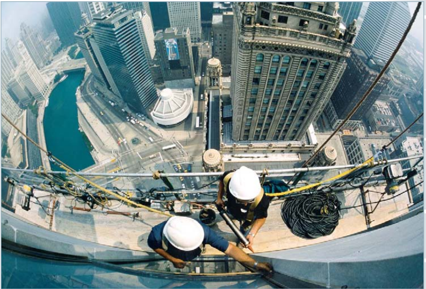
Flying high over Wacker Drive in downtown Chicago, inspectors with Western Waterproofing Co., Inc. work on a building's façade per Chicago's façade inspection ordinance.
