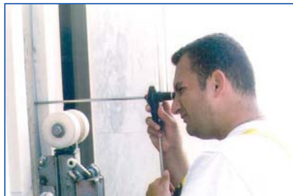
Figure 3 – A fiber optic borescope is used to view inside a building façade. Borescopes require small holes in building façades in order to peek inside the wall system.
