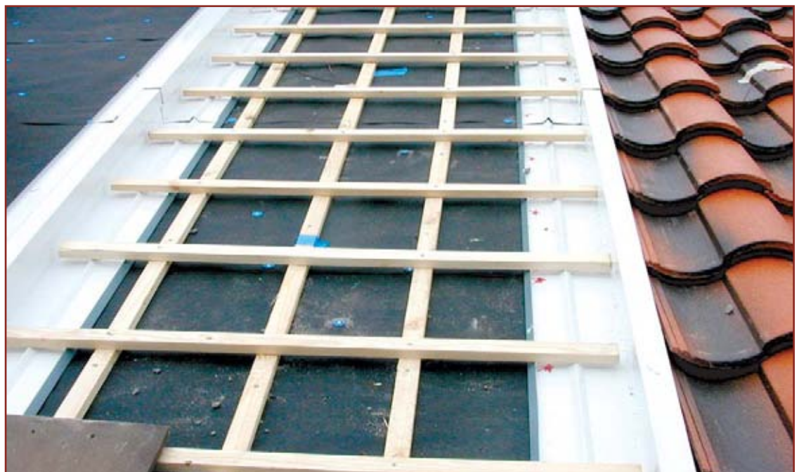
Figure 3 – Construction of the roof deck showing battens and counter-battens for attaching the slate tile. The parapets are used to limit airflow on the underside of the tile to within a given test roof.
