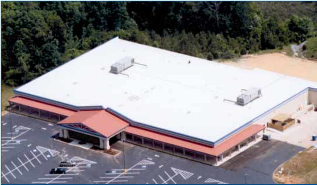
Photo 4 – Cool roofing systems are especially effective on low-rise buildings with large roof areas. Potential energy savings during the hot Mississippi summer months helped convince the Grenada Medical Complex in Grenada, Mississippi to install a recyclable, high-performance thermoplastic cool roofing system covering 69,474 square feet. (Photo courtesy of Duro-Last Roofing, Inc.)
