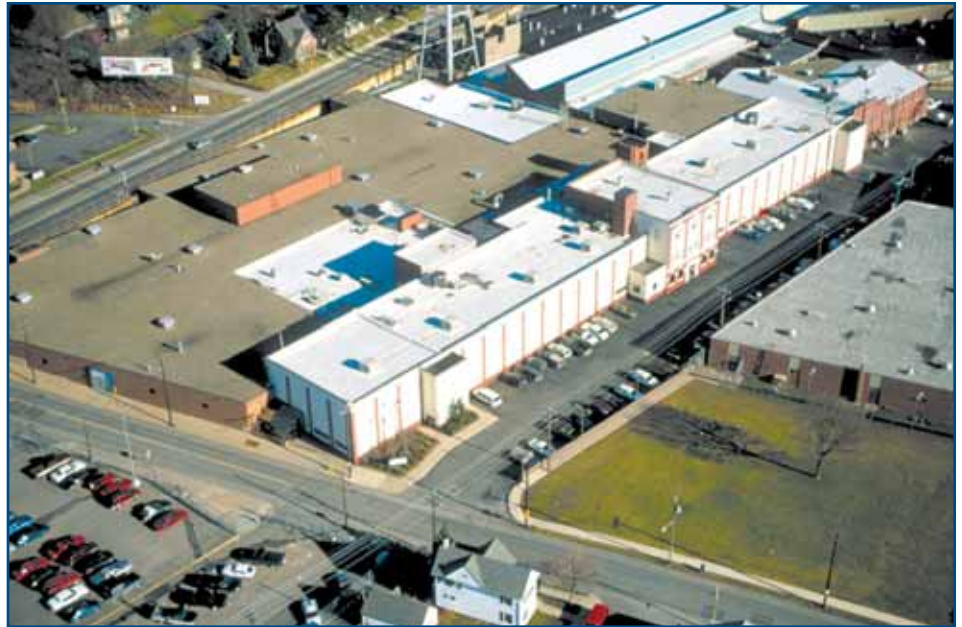
Photo 6 – High-performance roofing systems moderate indoor temperatures, even in buildings that are not fully air-conditioned at all times, such as the Textron manufacturing facility in Williamsport, Pennsylvania. Various studies have shown a direct relationship among thermal comfort, overall mental concentration, and manual work rates. (Photo courtesy of Duro-Last Roofing, Inc.)
