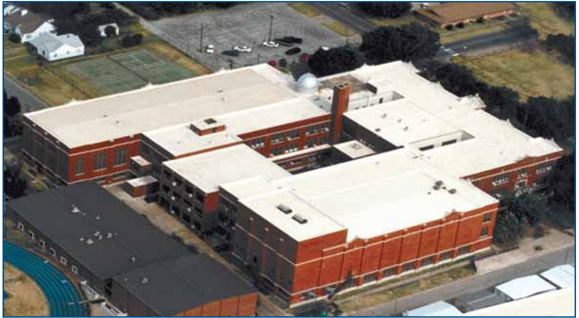
Photo 3 – According to roofing contractor Rod Heitfield, owner and president of Heritage Roofing Systems in Enid, Oklahoma, energy savings from the cool roofs installed in several other district schools were so great that they virtually paid for the entire 81,803-square-foot PVC cool roofing system protecting Enid High School. (Photo courtesy of Duro-Last Roofing, Inc.)
