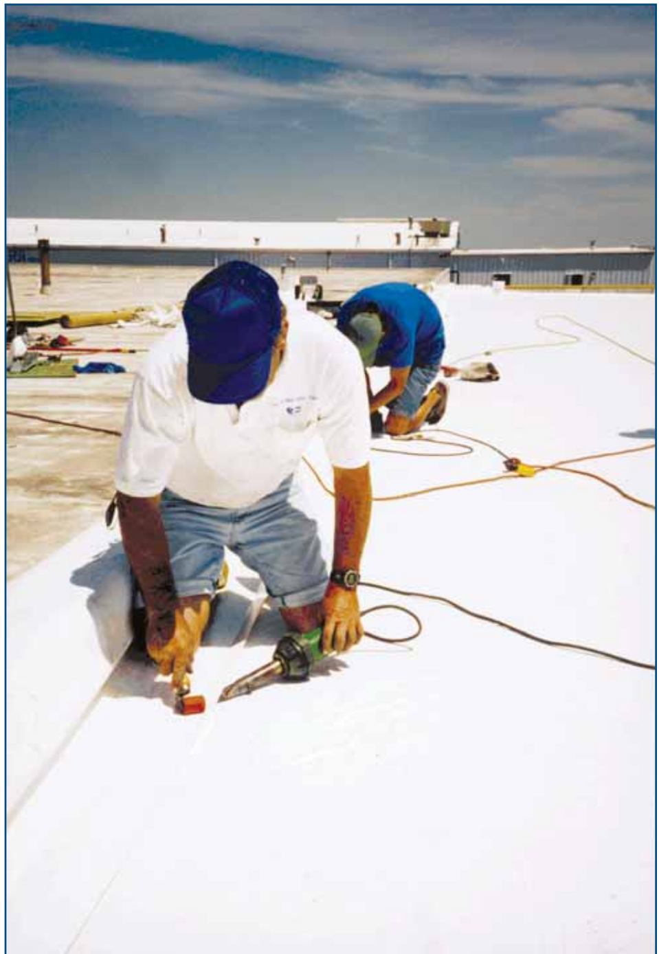
Photo 2 – By the late 1990s, cool roofing was the “hottest” trend in commercial roofing, and white thermoplastic single-plies began a sustained run as the fastest-growing category of commercial roofing systems. (Photo courtesy of Duro-Last Roofing, Inc.)
