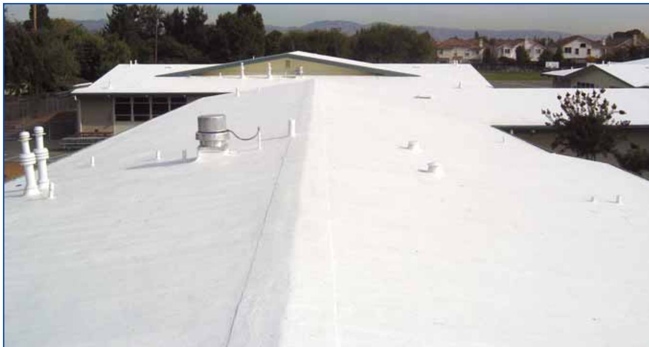
Photo 5 – Field-applied coating on a mineral-surfaced cap sheet.
