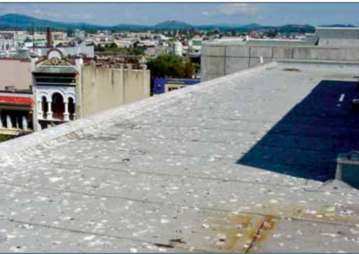
Photo 2 – The amount of fecal matter and damage discovered on the first site visit was quite astonishing... and the smell wasn't great either!
