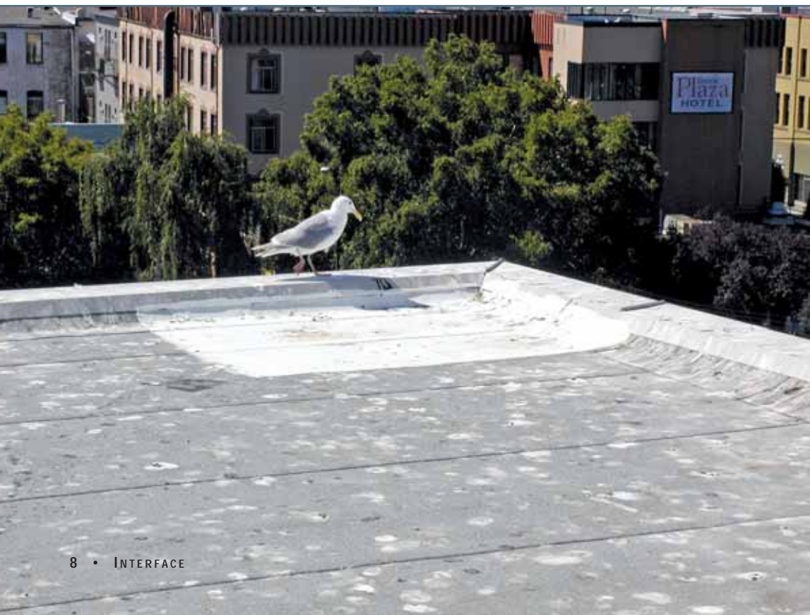
Photo 5 – One of the attempts to “fix” the problem was an elastomeric coating. As demonstrated, the birds loved it. This particular coating proved ineffective.
