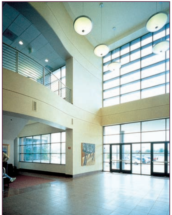
The use of curtain wall, such as at Empire College in Saratoga Springs, New York, is one way to bring natural light into a building.
