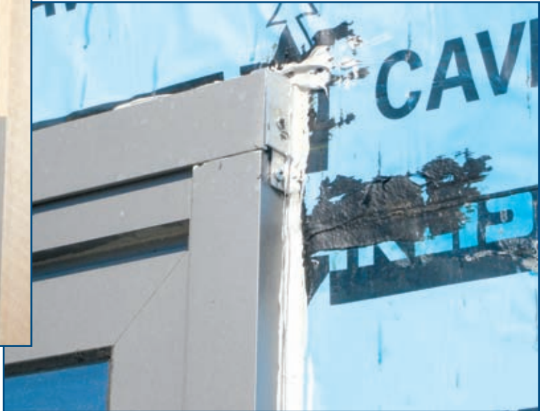
Photo 5 – Large end cap installed at ends of the head receptor.
