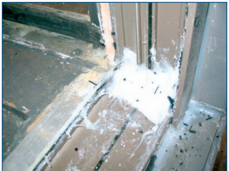
Photo 6 – Extremely heavy corner seal.
