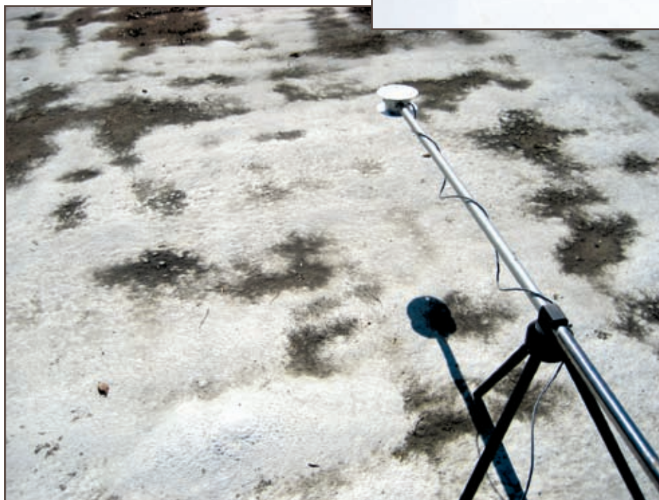
Photo 4 – SPF in Iowa, 3 years old, urethane/acrylic coating.
