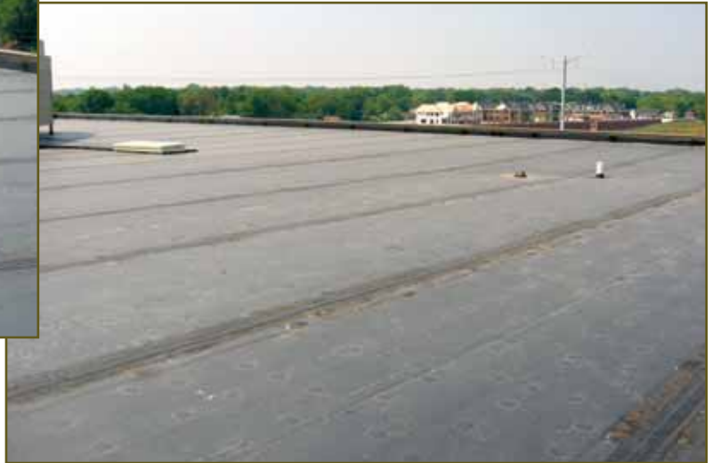
Photo 5 – This three-year-old, 90-mil EPDM roof, designed to FM 1-120 standards, is well on its way to achieving long-term service life (a minimum of 30 years). (Photo by Tom Hutchinson.)
