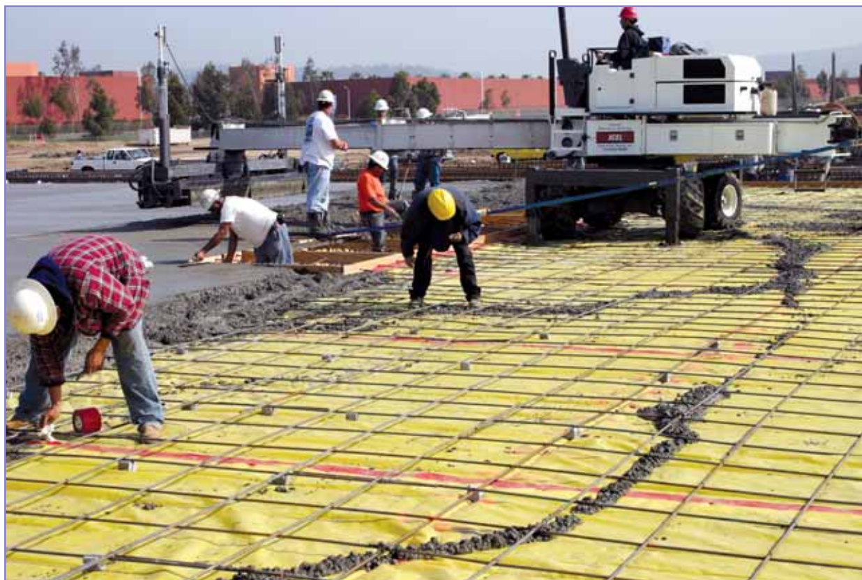
Low-permeance, below-slab vapor barrier
