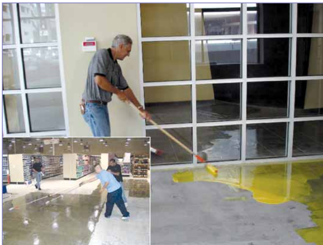
Application of topical moisture mitigation treatments
