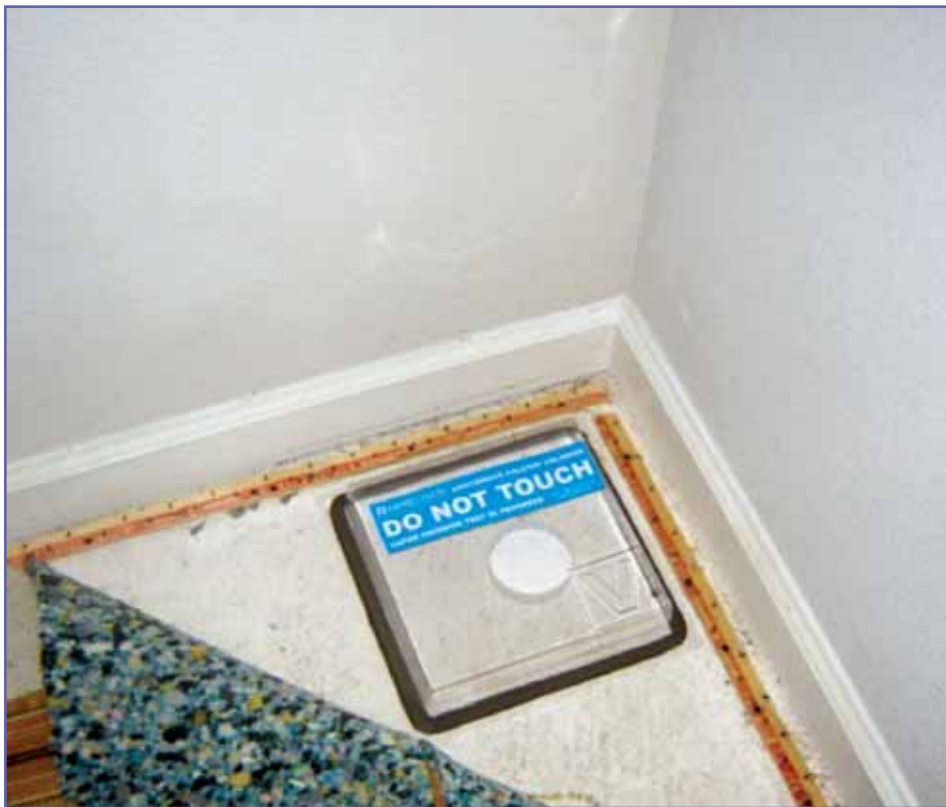
Photo 1 – Calcium chloride vapor emission test dome installed at concrete floor slab
