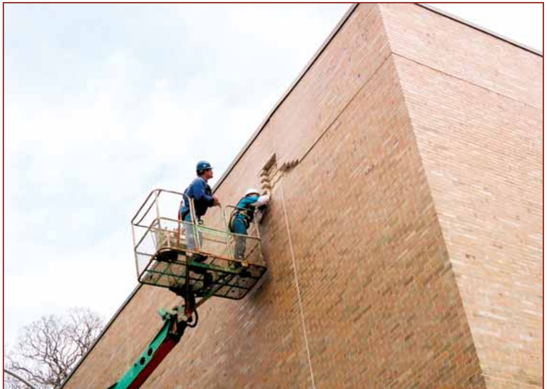
A masonry inspection opening
