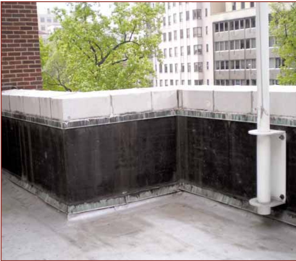
Roof run up the back of a parapet wall that created damage to the terra cotta cornice.
