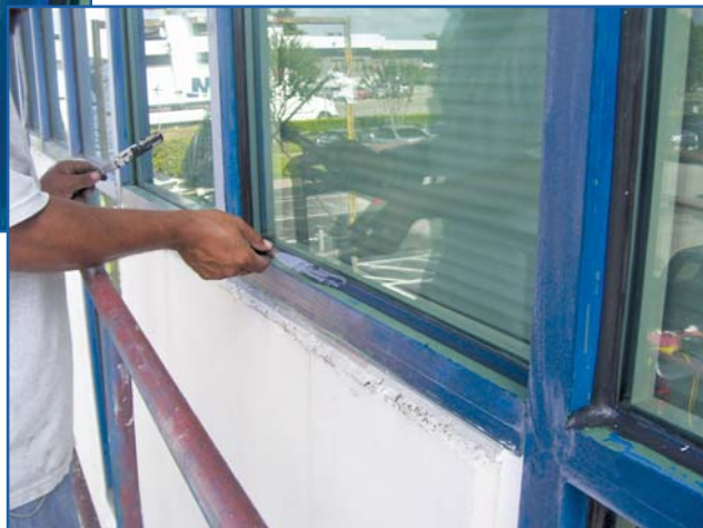
Figure 7 – Tooling sealant.
