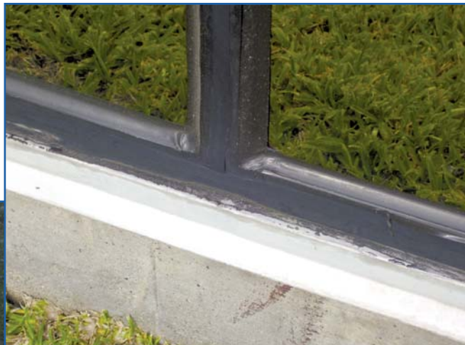
Figure 11 – Wet-sealed lockstrip.
