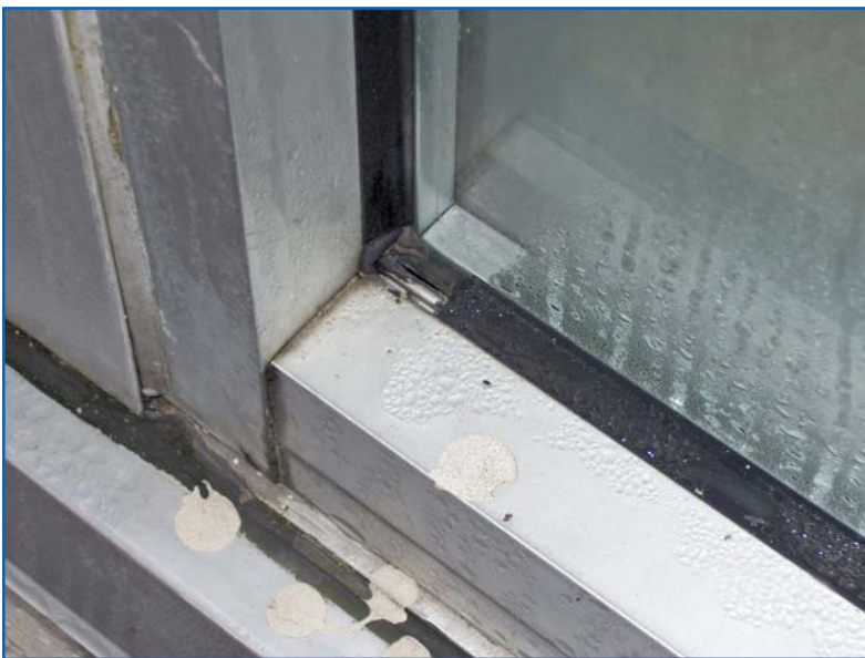
Figure 1 – Short gasket at corner of frame.
