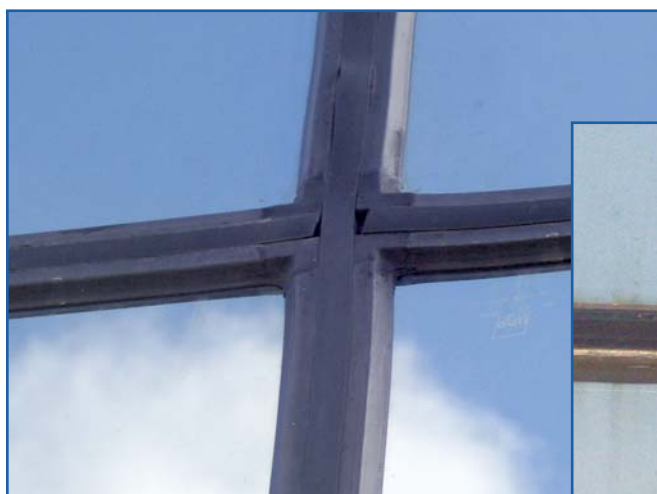
Figure 12 – Lock-strip gasket corner.
