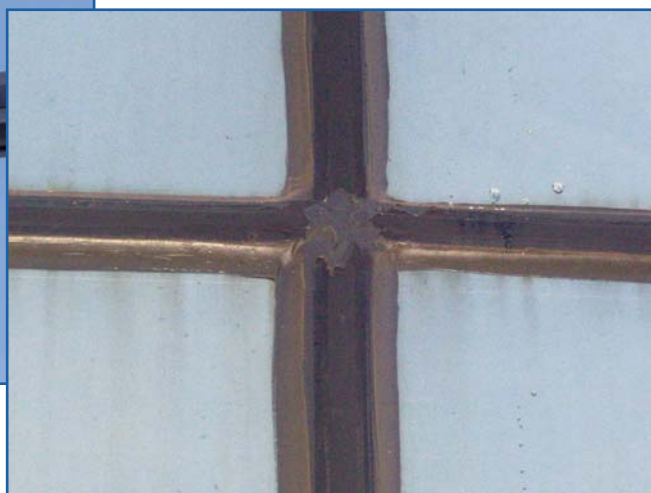
Figure 13 – Wet seal of lock-strip gasket.
