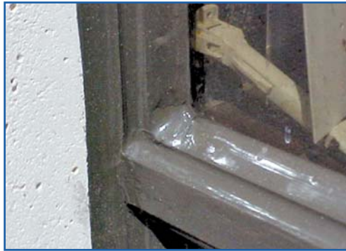
Figure 15 – Installed wet seal at window frame.
