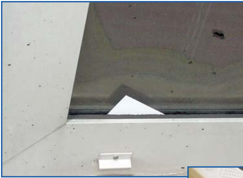
Figure 3 – Loose gasket.
