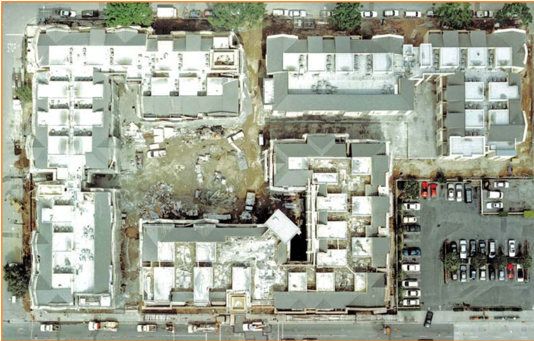
Photo 2 – Trammell Crow Residential project in Pasadena, California, seen from the air.
