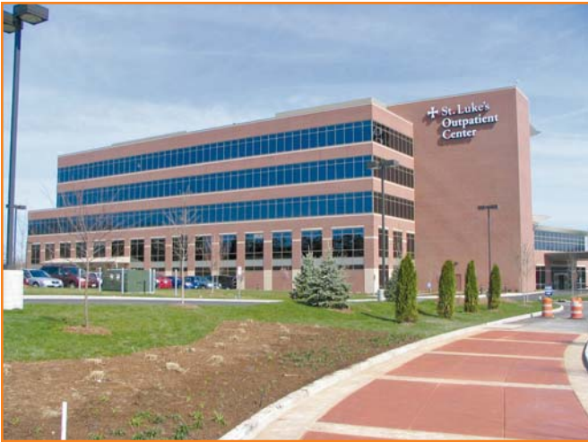
Photo 1 – Front of St. Luke's Outpatient Center.
