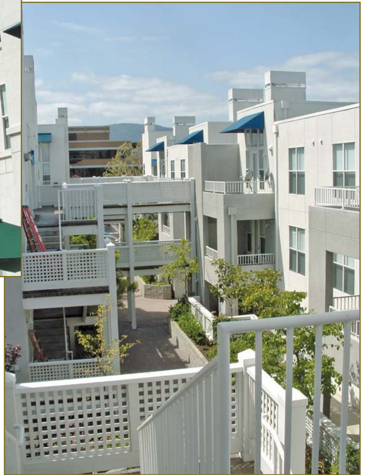
Photo 2 – Instead, the majority of the qualitative testing was carried out at the more readily accessible central courtyard.
