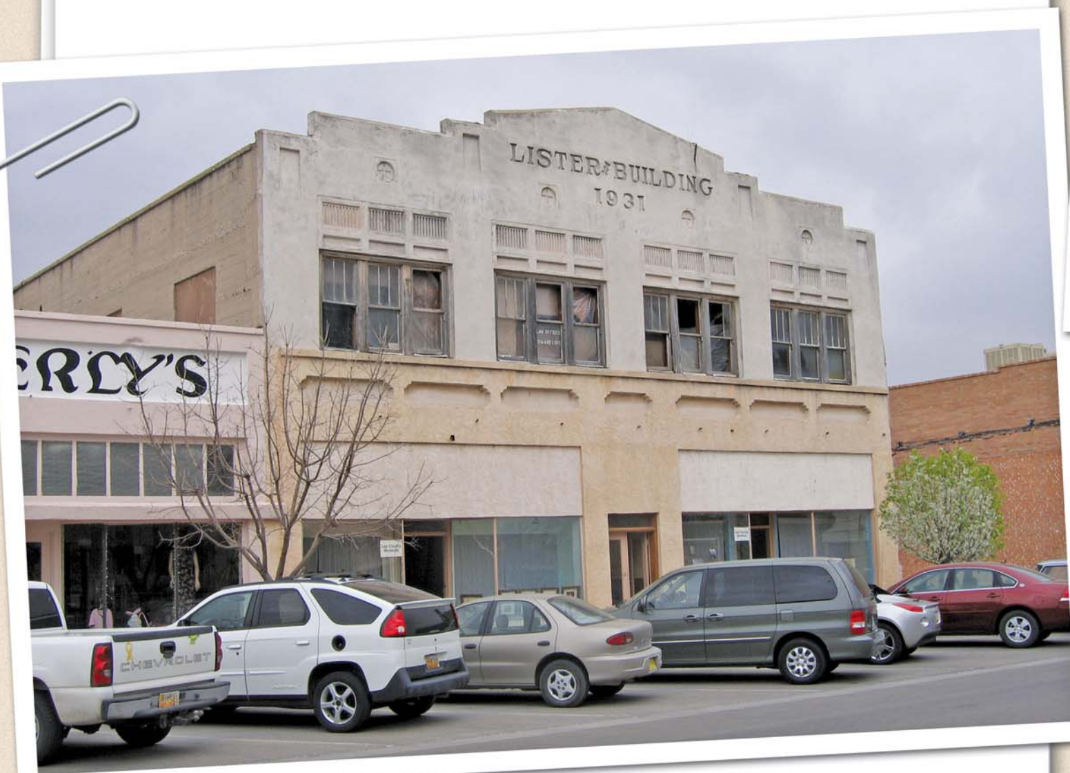
Built in 1931, the Lister Building in Lovington, NM, features a decorative façade that includes parapet walls ranging from 3 to 7 ft high.
