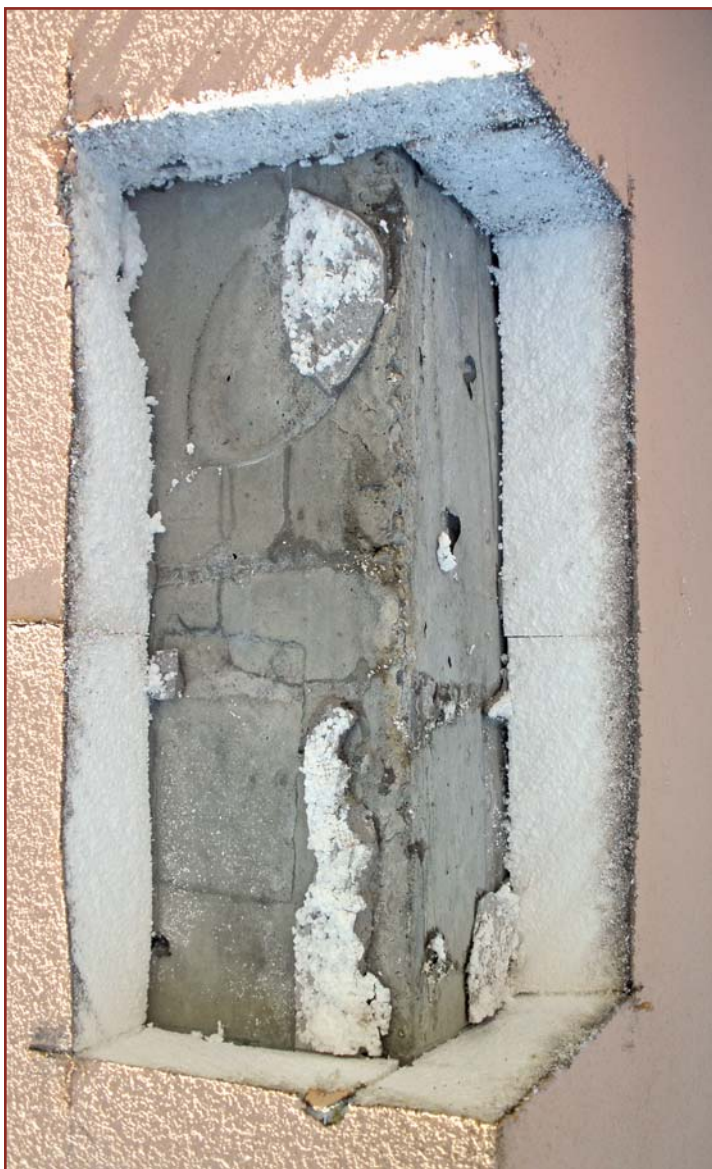
Photo 1 – Test opening at EIFS-clad wall.
