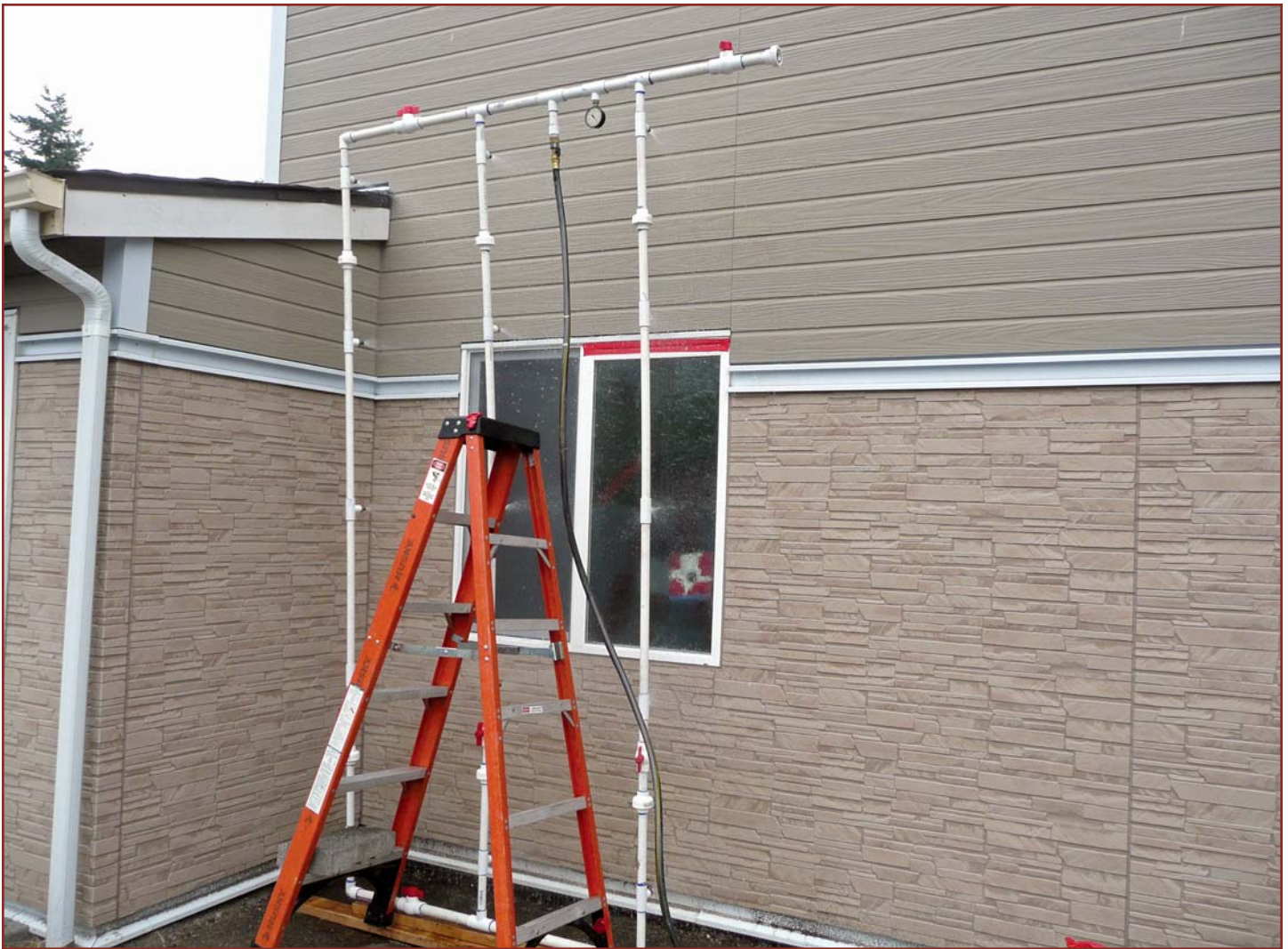
Photo 2 – Field testing of suspect window installation.
