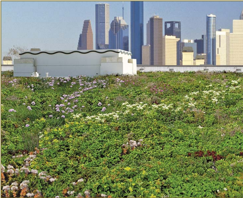
SPRI and the Dept. of Energy have jointly funded a program to quantify the energy savings associated with various types of vegetated roof systems. (Photo courtesy of GAF Materials Corporation, Wayne, NJ.)
