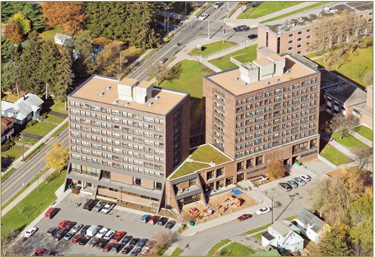
The State University of New York at Cortland recently gave this green roof center stage. In reaction to a code change put into the International Code Council (ICC) stating all vegetative roof systems must undergo wind and fire testing, standards are in development to address these criteria. (Photo courtesy of Siplast Inc., Irving, TX.)
