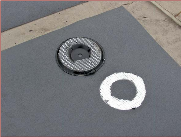
Photo 6 – The tool must be calibrated based on the ambient temperature to provide an optimal bond. A properly bonded plate will provide total, even, and consistent fusion of the membrane.
