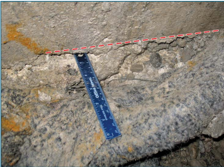
Figure 9 – Channel-like cavity in footing between smooth side (above dotted line) and bulge.
