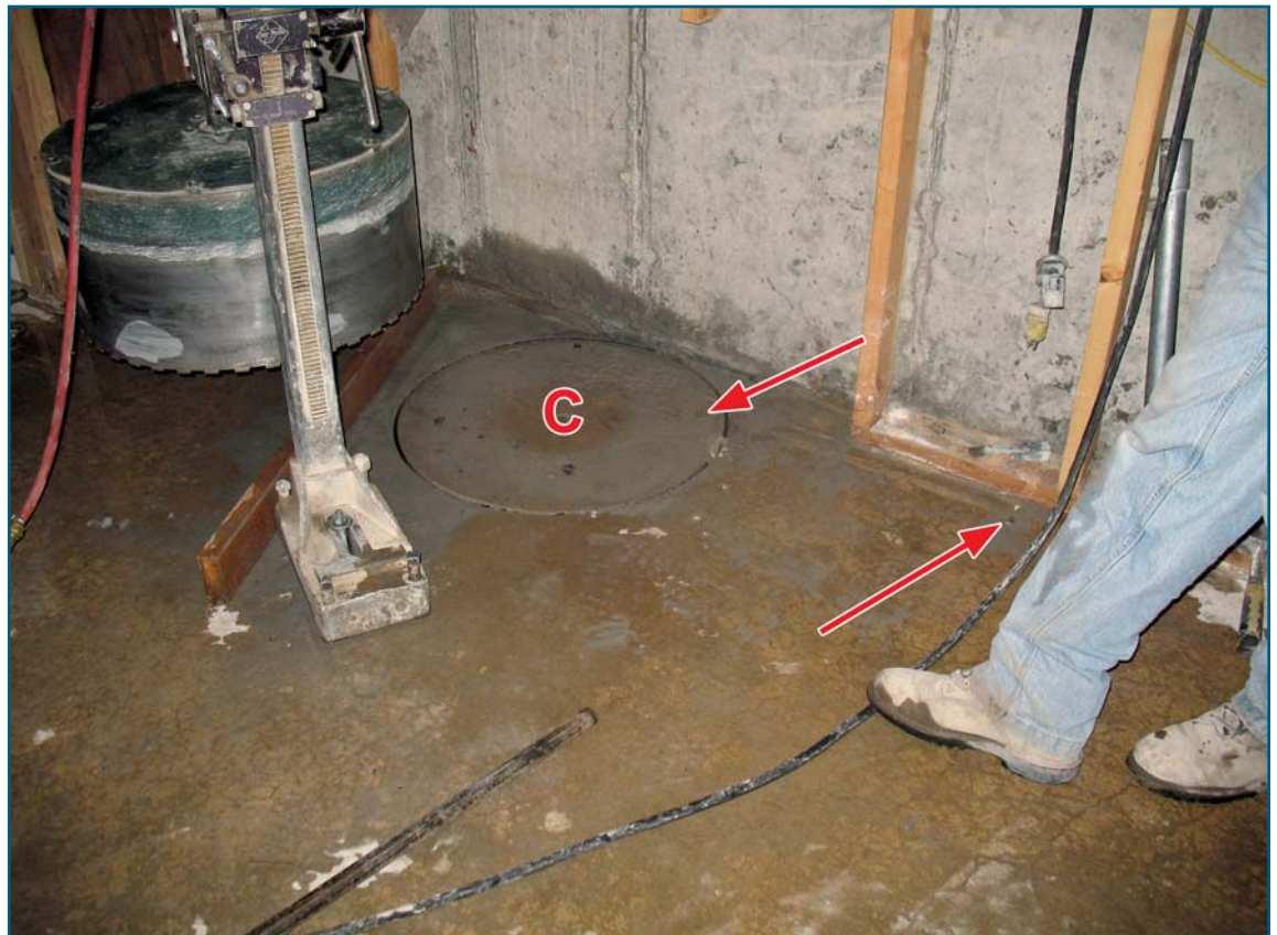
Figure 4 – Locations of core (C) and grout injection holes (at arrows).
