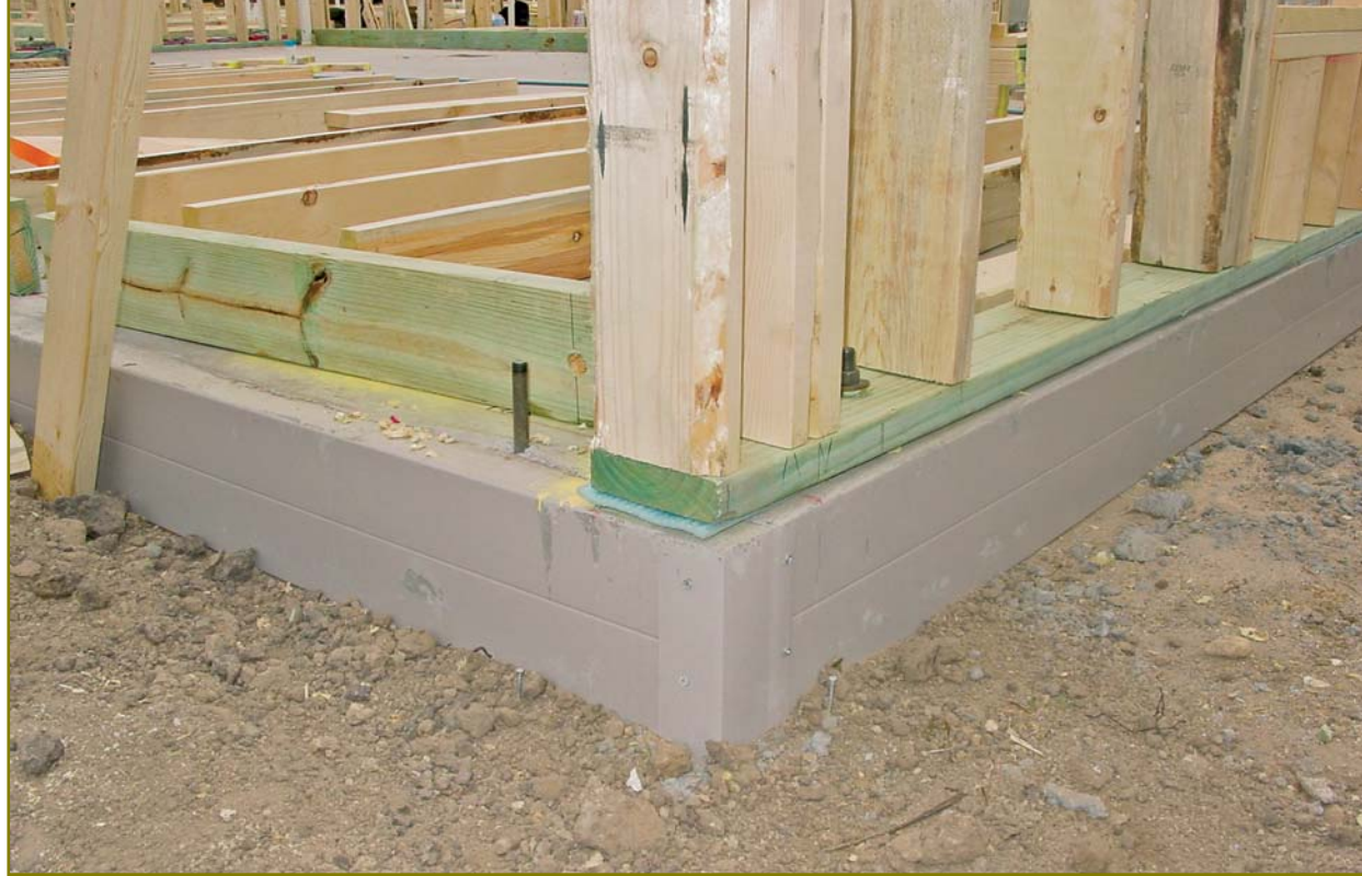
Figure 2 – EnergyEdge® remains in place as part of the foundation, leaving a finished and insulated slab edge with an R-10 thermal resistance value, meeting International Energy Conservation Code (IECC) requirements.
