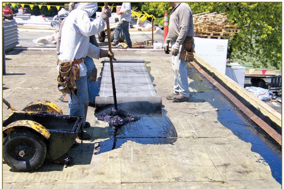
Photo 7 – Modified bitumen is installed directly on the stone-wool insulation in hot asphalt.
