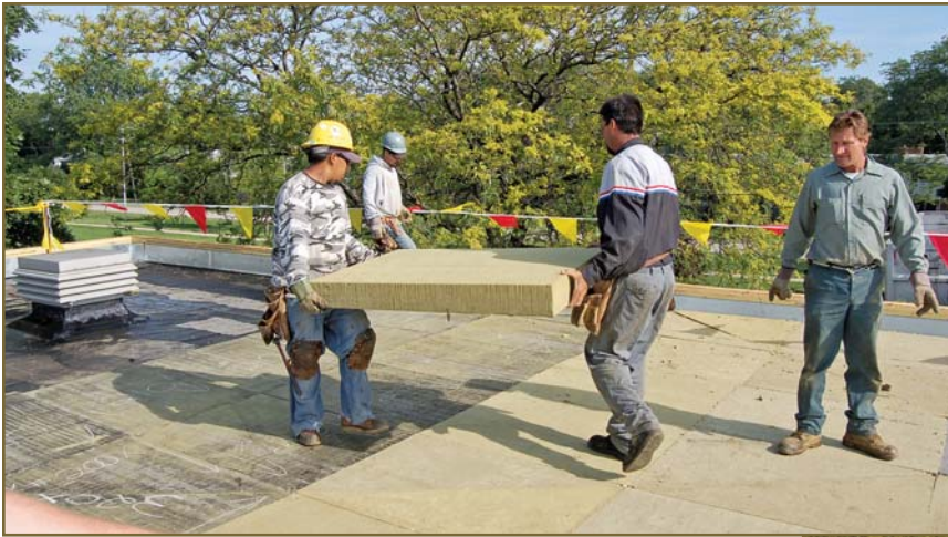
Photo 5 – Full-thickness stone wool panels are set into place.
