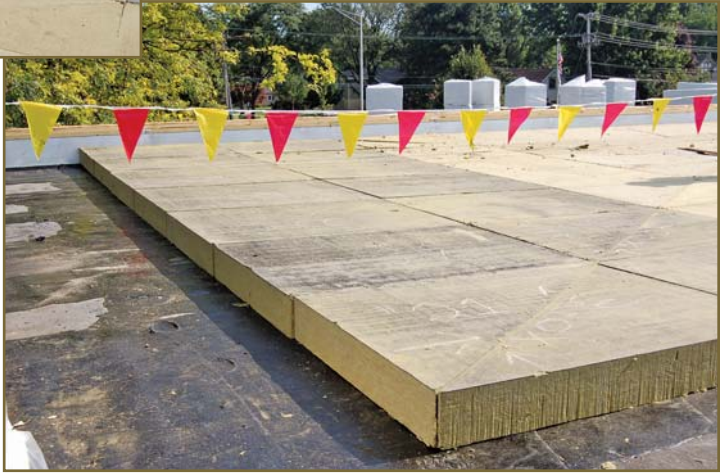
Photo 6 – Tapered stone wool panels set in hot asphalt.
