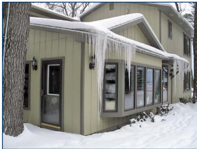
Figure 1 - Typical ice dam.
