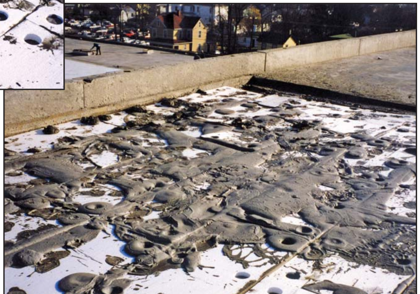
Figures 1 and 2 — What may first appear to be a random mess is instead a quite viable roof deck system. Here, polystyrene boards are situated into wet LWIC. The polystyrene provides the bulk of the R-value, while holes and slots in the boards provide a “keying-in” of these materials.
