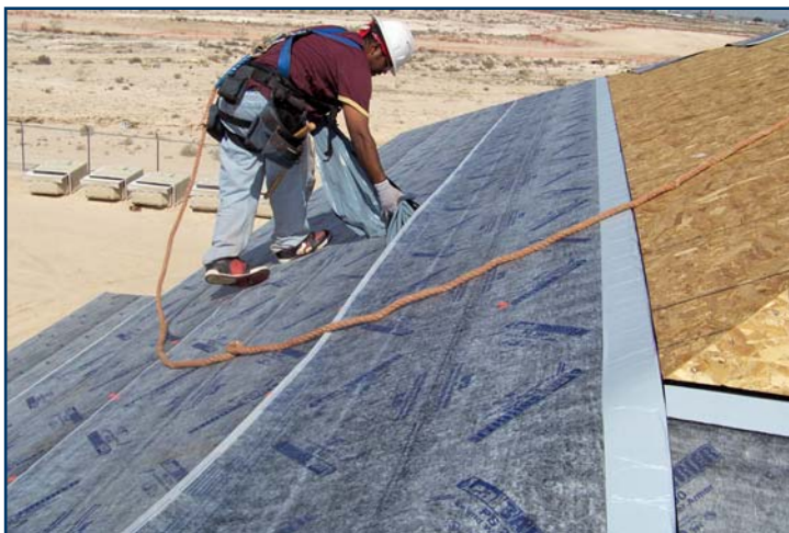
Figure 3 – The PS200HT self-adhering underlayment has fiberglass reinforcement and high temperature resistance. It is suitable for metal, tile, or shingle applications.
