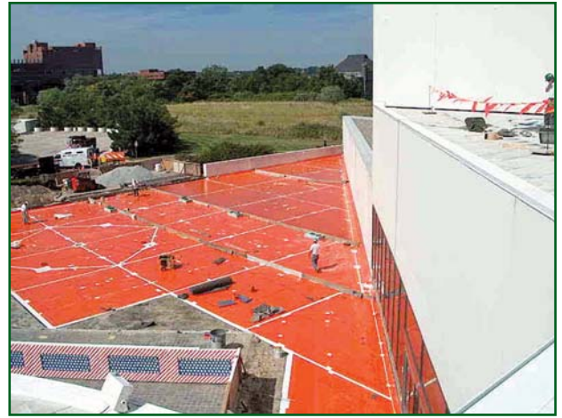
Photo 9 – Thermoplastic waterproofing membrane/grid system.
