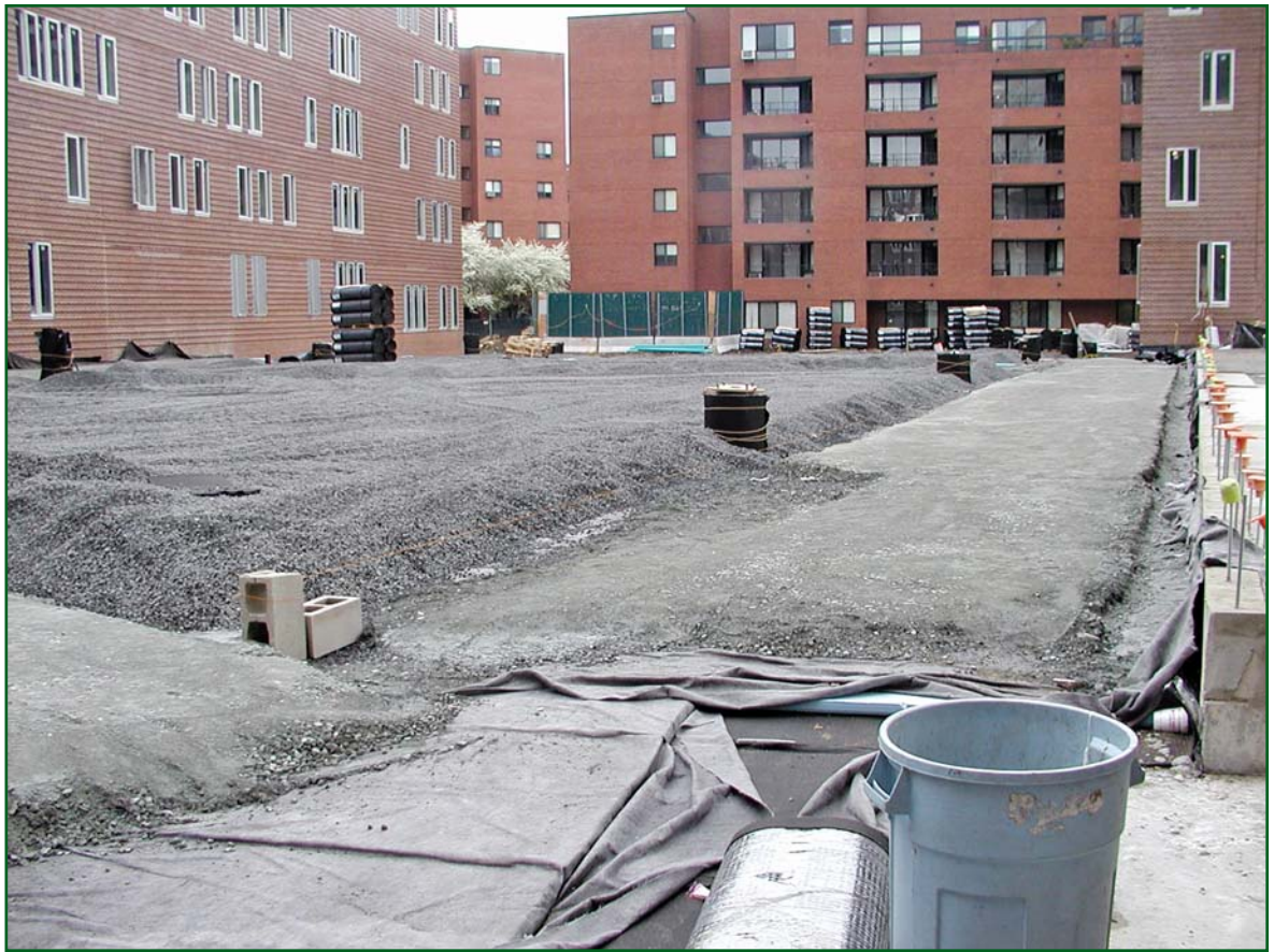
Photo 8 – Various media layers being installed.
