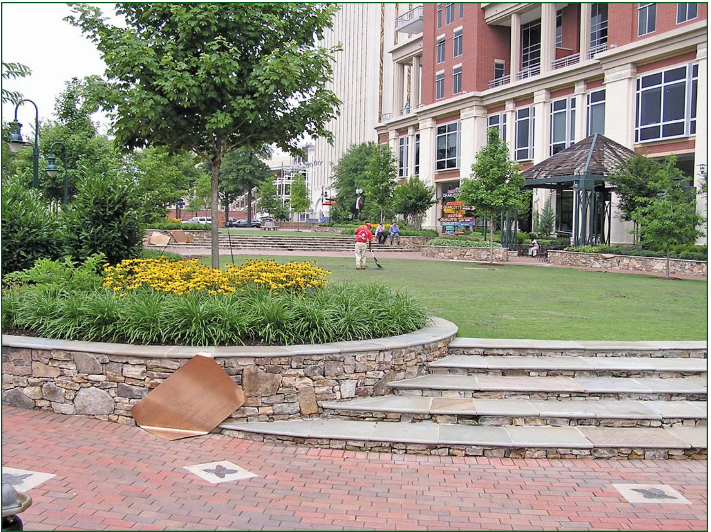
Photo 3 – Plaza/green roof assembly.
