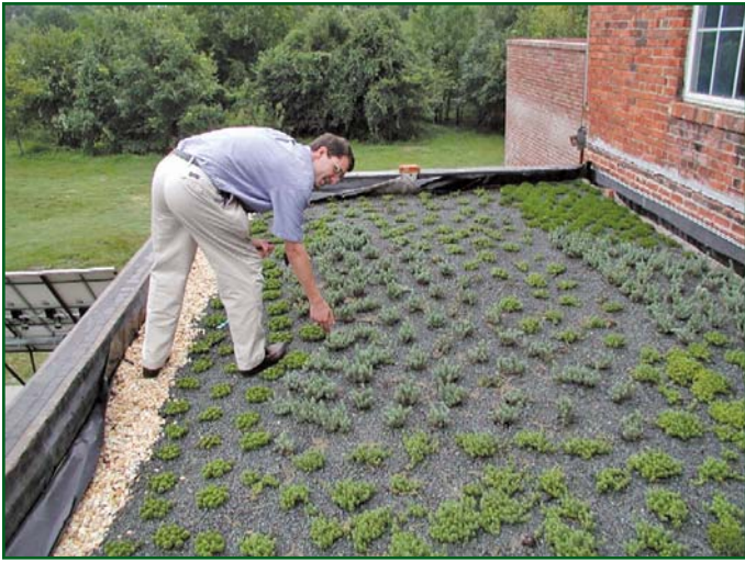
Photo 4 – Installation of media and planting.
