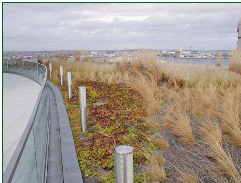
Photo 1 – Garden roof on a high-rise building in Boston, MA.
